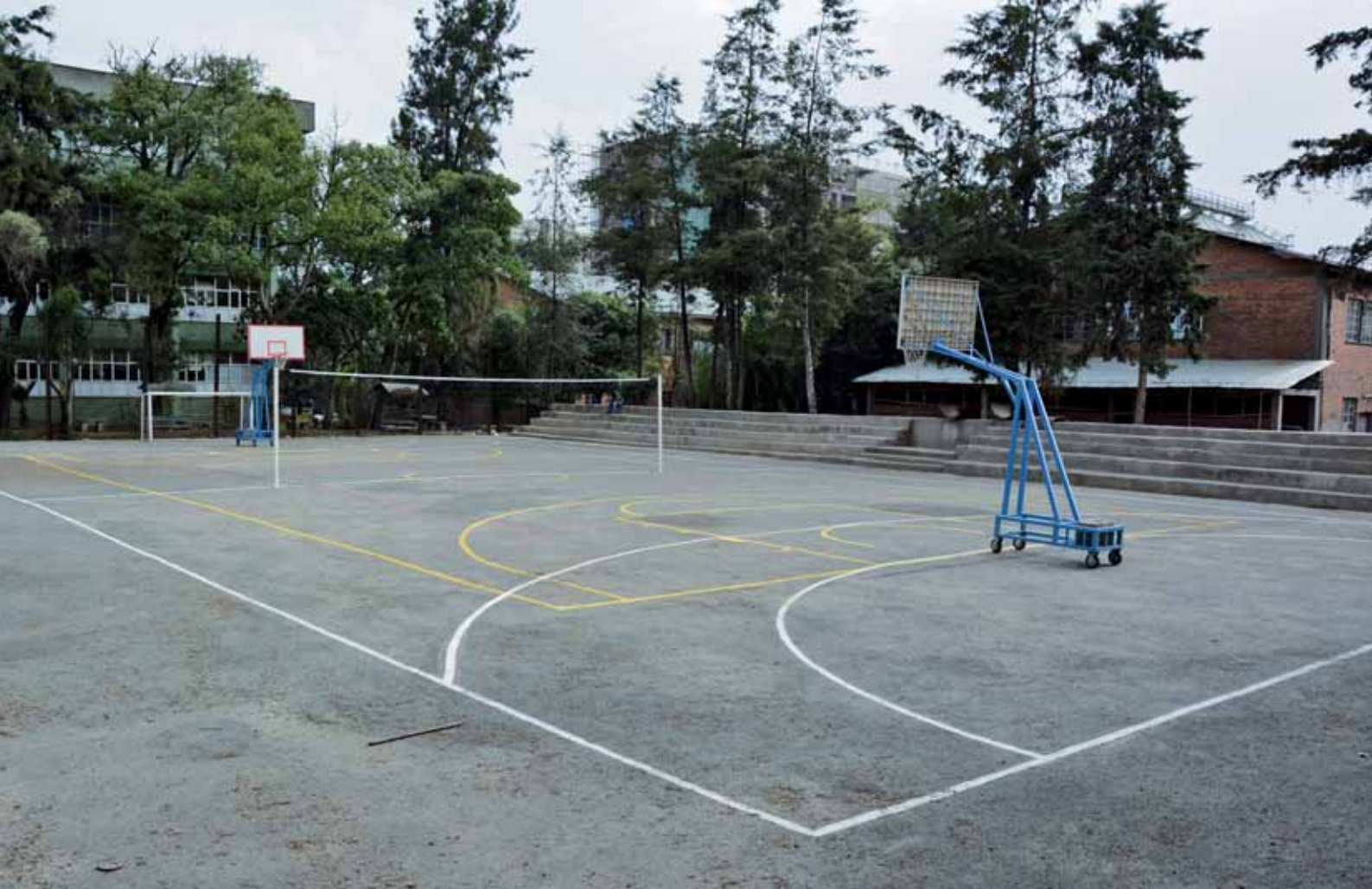
Asphalt sports ground at Tegere-Id Polytechnic College in Ethiopia | © GIZ/Addisalem Nega
