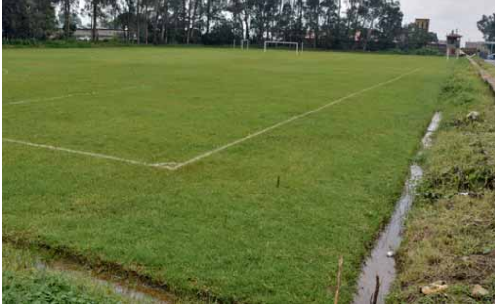
Natural earth channel (drainage type 1) filled with excess water at Entoto Polytechnic College in Addis Ababa, Ethiopia | © Addisalem Nega
