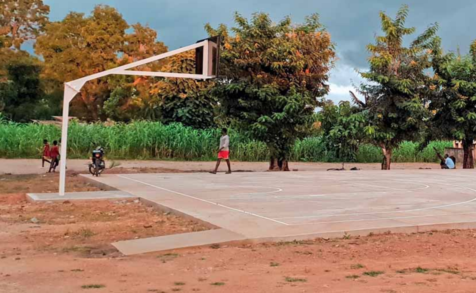
Asphalt sports ground with ramps ensure accessibility, Togo | © GIZ/Akimbi Akpado
